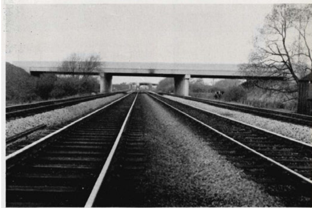
"Eight minutes to place a beam . . . B.R. allowed the contractors to place 3 beams a day."
